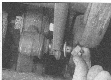
7.8a Locate the balljoint in the axle, and refit its retaining nut and washer
